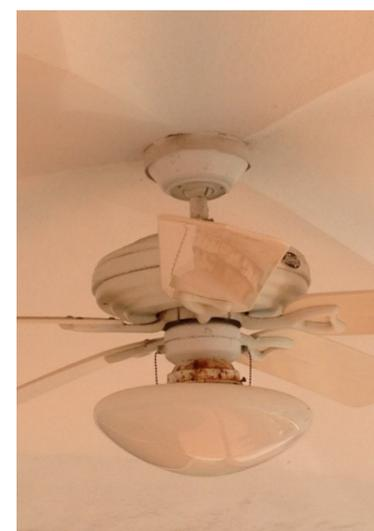
⇒ Rust forming on the fan housing above the light
